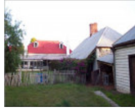
Exford Homestead - rear elevation
