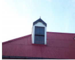
Dormer window (front elevation of Homestead)
