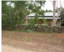
Dry Stone Wall L156
