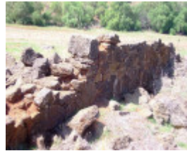
Bluestone ruins alongside the Toolern Creek
