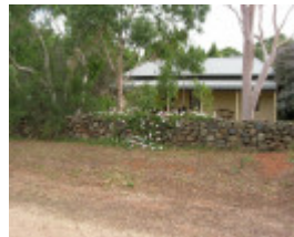
Dry Stone Wall L156
