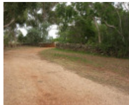
Dry Stone Wall L156
