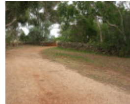
Dry Stone Wall L156
