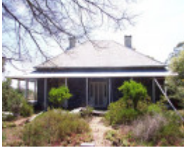
Strathtulloh Homestead - Greigs Road MELTON SOUTH, MELTON SHIRE
