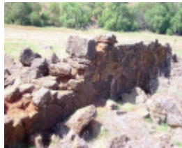
Bluestone ruins alongside the Toolern Creek
