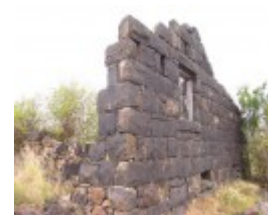
Deanside - Bluestone Ruin
