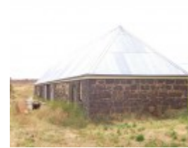
Deanside - Stables Building
