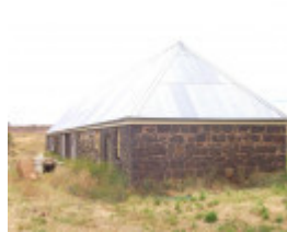
Deanside - Stables Building
