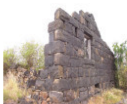
Deanside - Bluestone Ruin
