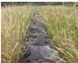
Deanside - Dry Stone Wall
