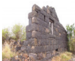
Deanside - Bluestone Ruin
