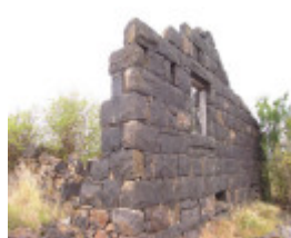
Deanside - Bluestone Ruin
