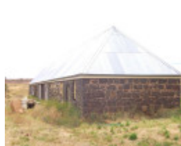
Deanside - Stables Building
