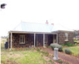
Deanside - Managers House
