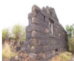
Deanside - Bluestone Ruin
