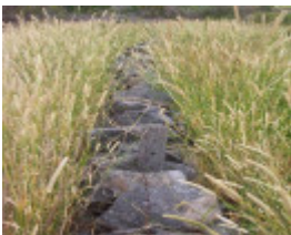
Deanside - Dry Stone Wall
