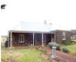
Deanside - Managers House
