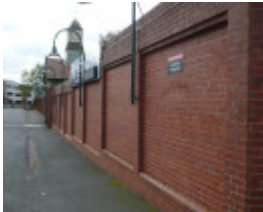
McPherson Street wall looking north
