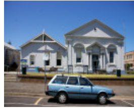
H543 orderly room gun room
