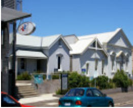
H543 orderly room residence kepler st1
