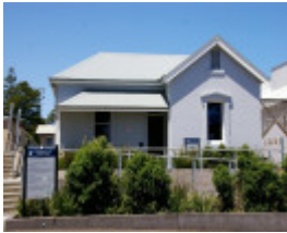
H543 orderly room residence
