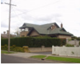
13 Retreat Road, Newtown - Exterior
