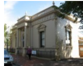
Mechanics Institute_Hamilton_1872 facade_KJ_April 09
