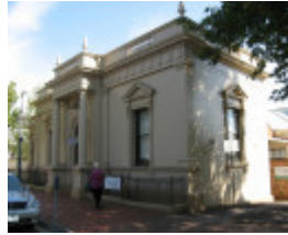
Mechanics Institute_Hamilton_1872 facade_KJ_April 09
