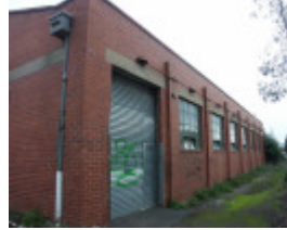
Factory, north (rear) elevation
