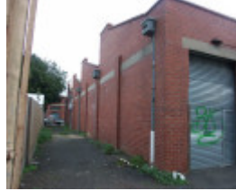
Factory, east (side) elevation
