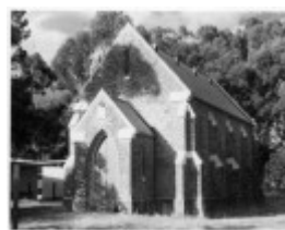
St Stephen's Anglican Church John Collins 1982 SLV
