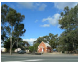
St Stephen's Anglican Church - front aspect from road 2008
