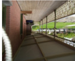
13 Stephen Street, Newtown - Photo 3 - On Verandah
