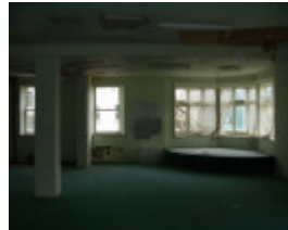
13 Stephen Street, Newtown - Photo 5 - Interior
