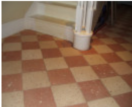
13 Stephen Street, Newtown - Photo 4 - Floor
