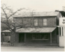
B2634 Old Brick Shop
