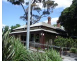
Domain former gardeners cottage Alexandra Gardens.JPG
