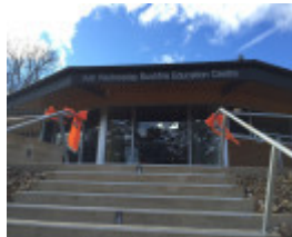
After Photograph - Reference F3896 2016
