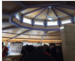
After Photograph - Reference F3896 2016
