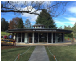
After Photograph - Reference F3896 2016
