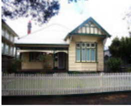
RICHMOND DAVISON STREET 35.jpg
