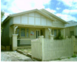
23 Ann Street, Geelong West
