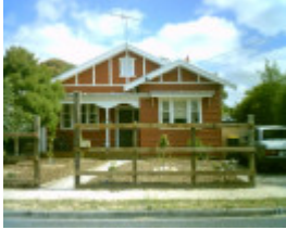
25 Ann Street, Geelong West
