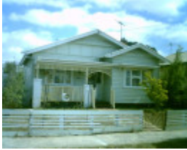
29 Ann Street, Geelong West
