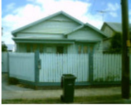
41 Ann Street, Geelong West
