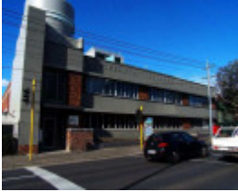
RICHMOND HODDLE STREET 129
