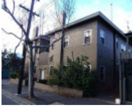
RICHMOND HODDLE STREET 141-143 Unit 1.jpg
