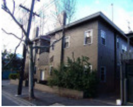
RICHMOND HODDLE STREET 141-143 Unit 1.jpg
