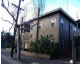
RICHMOND HODDLE STREET 141-143
