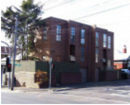
RICHMOND HODDLE STREET 147 Unit 1.jpg
