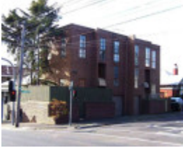
RICHMOND HODDLE STREET 147 Unit 1.jpg
