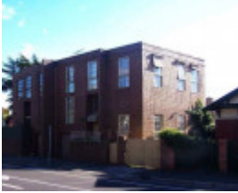
RICHMOND HODDLE STREET 147 Unit 2.jpg
