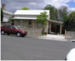
5 Arnott Street, Geelong West
