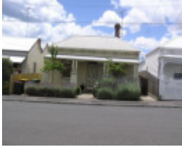
6 Arnott Street, Geelong West
