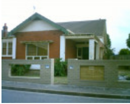
18 Askew Street, Geelong West
