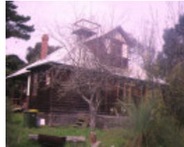
1 ballara glaneuse road point lonsdale rear elevation jun1995
