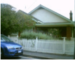
20 Askew Street, Geelong West
