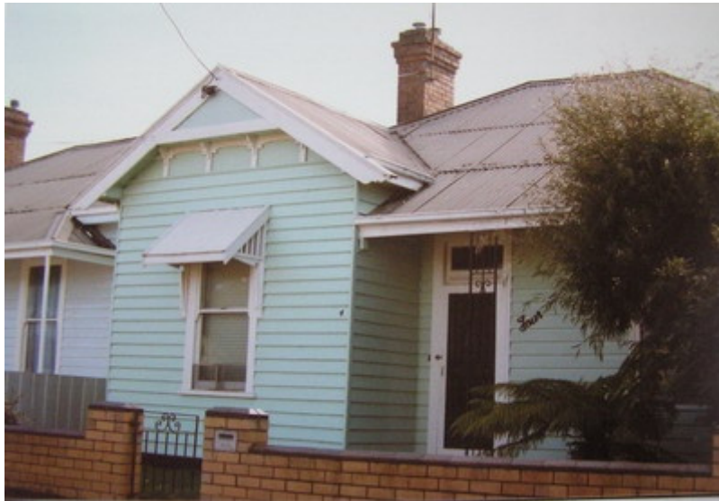
Source: Aitken, Honman & Huddle, 'City of Geelong West Urban Conservation Study', 1986.
