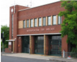
BRUNSWICK FIRE STATION AND FLATS SOHE 2008
