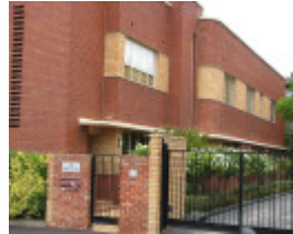
BRUNSWICK FIRE STATION AND FLATS SOHE 2008
