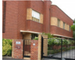
BRUNSWICK FIRE STATION AND FLATS SOHE 2008
