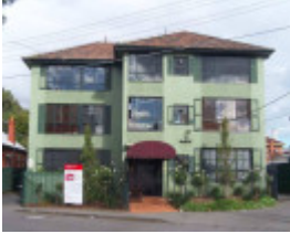
RICHMOND SMITH STREET 4 Unit 5.jpg
