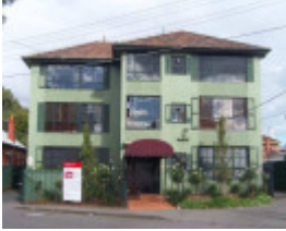
RICHMOND SMITH STREET 4 Unit 6.jpg
