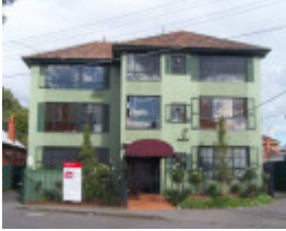
RICHMOND SMITH STREET 4 Unit 7.jpg
