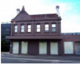
RICHMOND BURNLEY STREET 53.jpg
