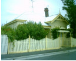
5 Catherine Street, Geelong West
