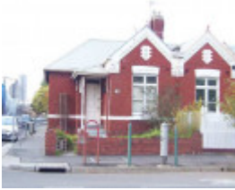
RICHMOND BURNLEY STREET 97.jpg
