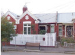
RICHMOND BURNLEY STREET 99.jpg
