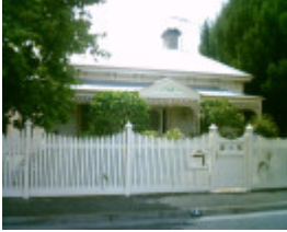
14 Catherine Street, Geelong West
