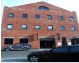
RICHMOND BROMHAM PLACE 8 Unit 4.jpg
