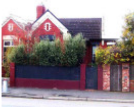
RICHMOND BURNLEY STREET 103.jpg
