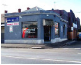
RICHMOND BURNLEY STREET 115.jpg
