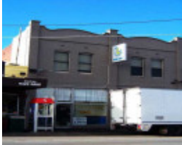
RICHMOND BURNLEY STREET 125.jpg
