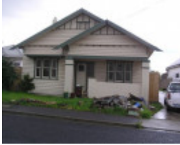
30 Clarence Street. Geelong West
