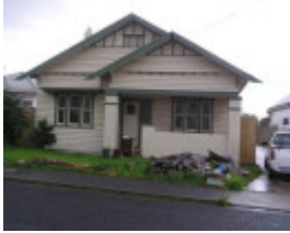
30 Clarence Street. Geelong West
