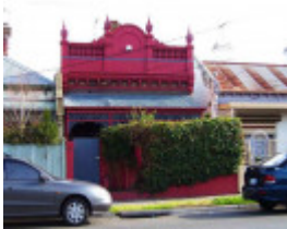
RICHMOND BURNLEY STREET 254.jpg
