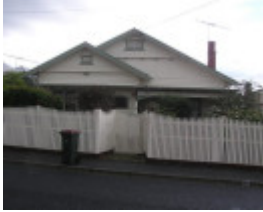
40 Clarence Street. Geelong West
