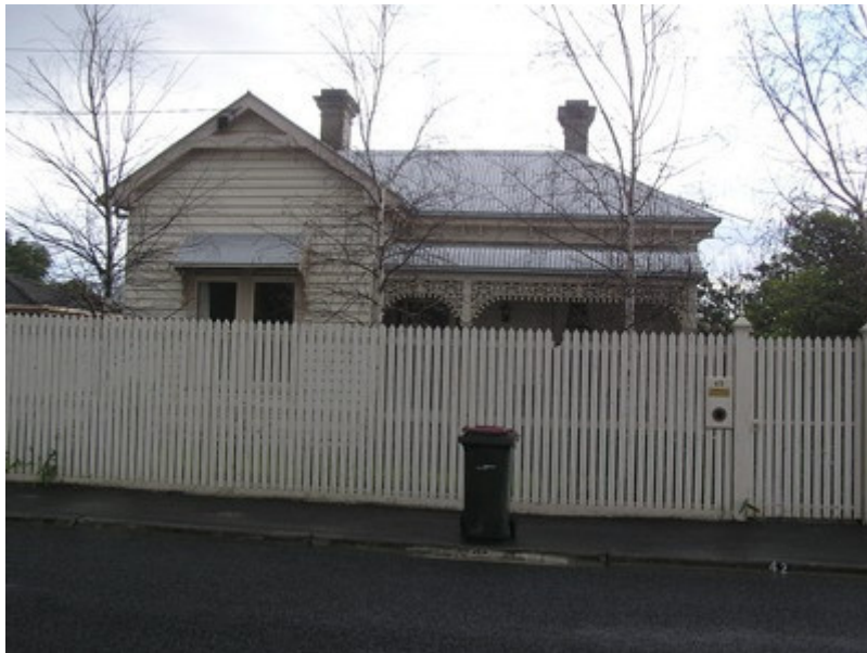
42 Clarence Street, Geelong West
