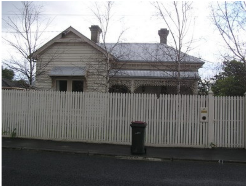
42 Clarence Street, Geelong West
