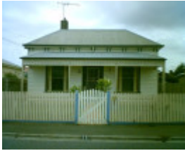
56 Clarence Street, Geelong West
