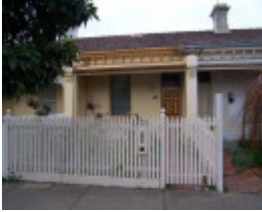
RICHMOND BURNLEY STREET 349.jpg
