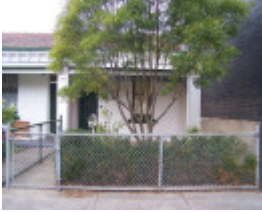
RICHMOND BURNLEY STREET 367.jpg
