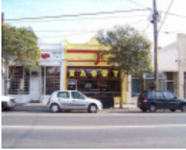
RICHMOND BURNLEY STREET 378.jpg
